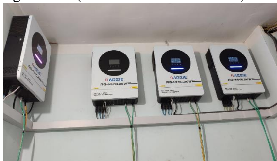
Figure 7. FES inverters and junction box installed in Mingbulok District Medical Association.
